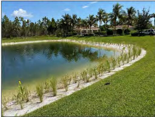
Figure 1. Vegetated Regraded Lake Bank. (Seabreeze Erosion Solutions, 2025)
