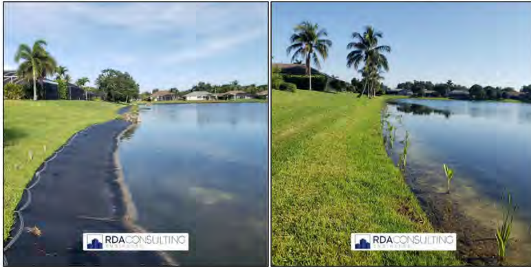
Figure 7. Erosion Control Wraps During and After. (RDA Consulting Engineers, 2026).
