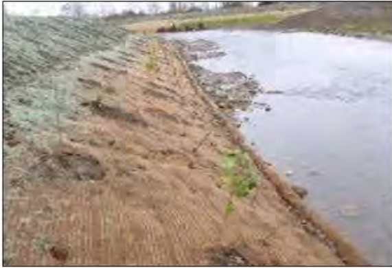
Figure 4. Biodegradable Erosion Control Mat. (Erosion Control Products, n.d.)
