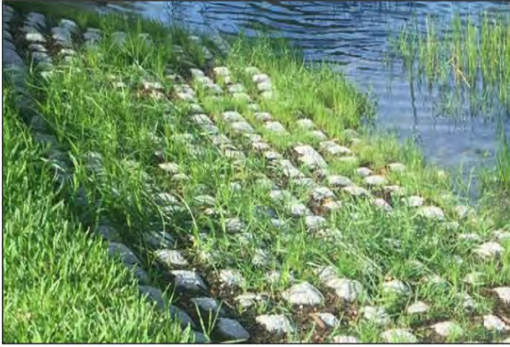
Figure 5. Vegetated Concrete Mat, Flexamat. (Seabreeze Erosion Solutions, n.d.)
